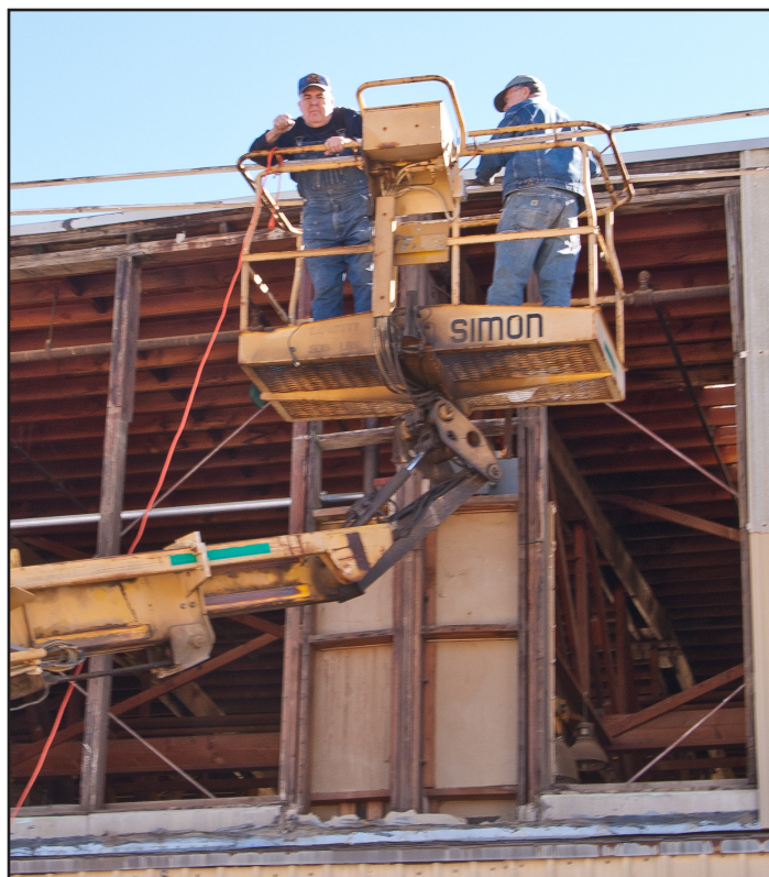
Recent high winds in Campo tore some panels off the side of the shop building. Larry Rose (L) and Frank Stites used the man lift to replace the panels. John Wright Photo
