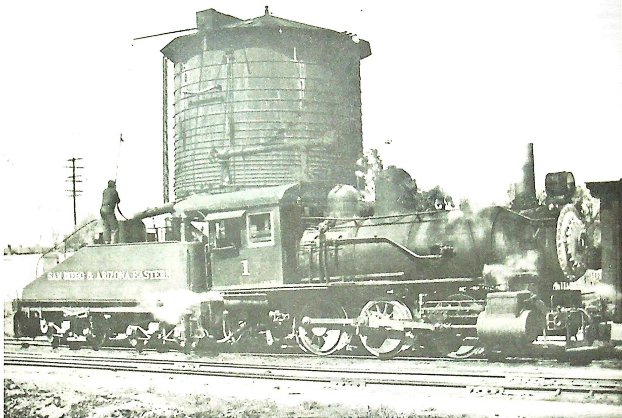
San Diego & Arizona Eastern Railway Co. Locomotive No. 1 in the San Diego yards, March 1948. (Eric Sanders)
