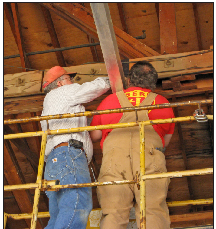
Frank Stites (L) and Rusty Hoar installing the safety rail in the overhead of the shop.
