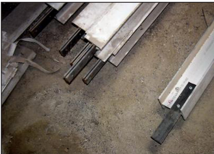
The rails prior to installation, showing the joint bracket.
