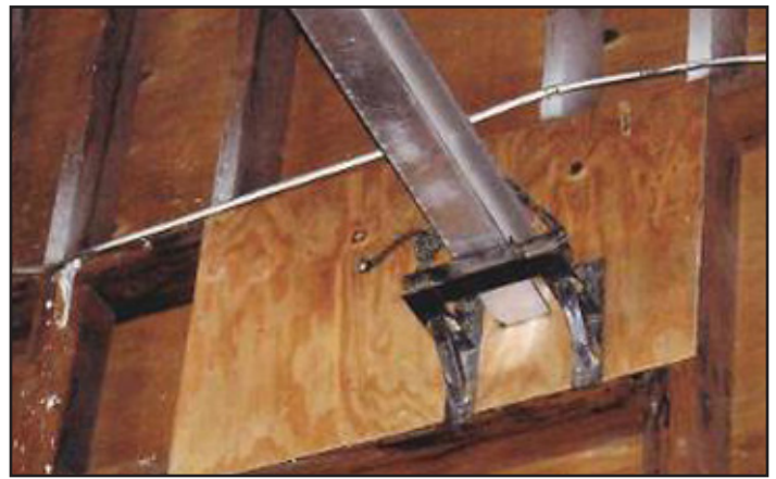
End view of the rail showing the mounting bracket at the ends of the building.
