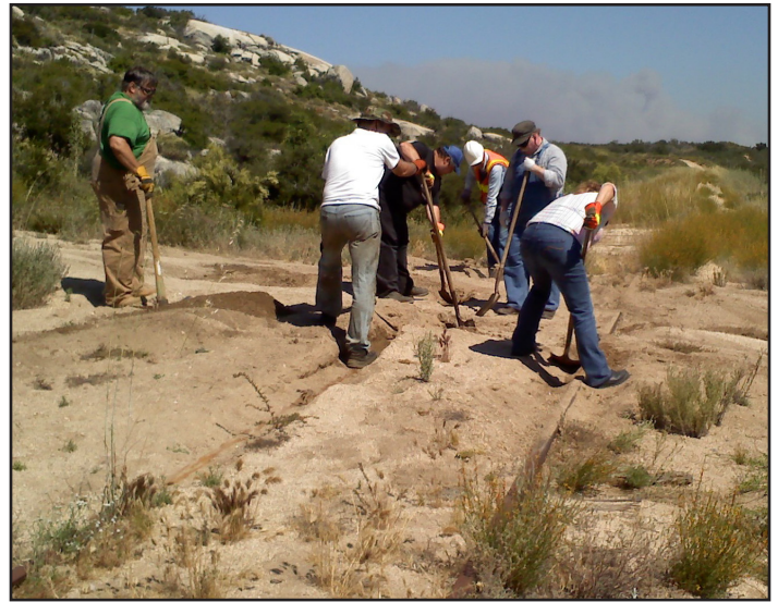
Clearing the track at Milepost 79.5. From Left: Rusty Hoar, John Shannon, Dave DiGiorgio, Rich Paulus, Ron Hyatt and Diana Hyatt. Photo By Cheryl Hoar
