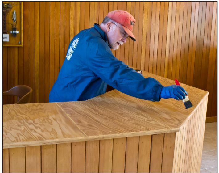
Frank Stites applies a coat of varnish to the top of the ticket counter.
