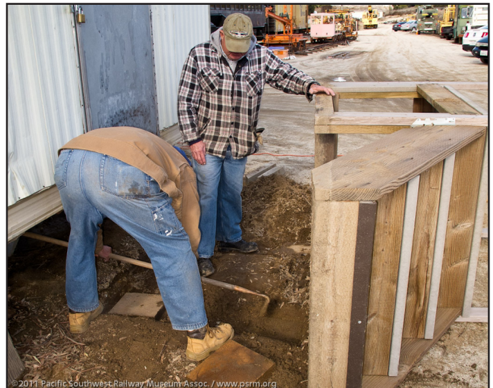
Larry Rose (left) and Seth Miller leveling the foundation and stairs of the operations trailer.
