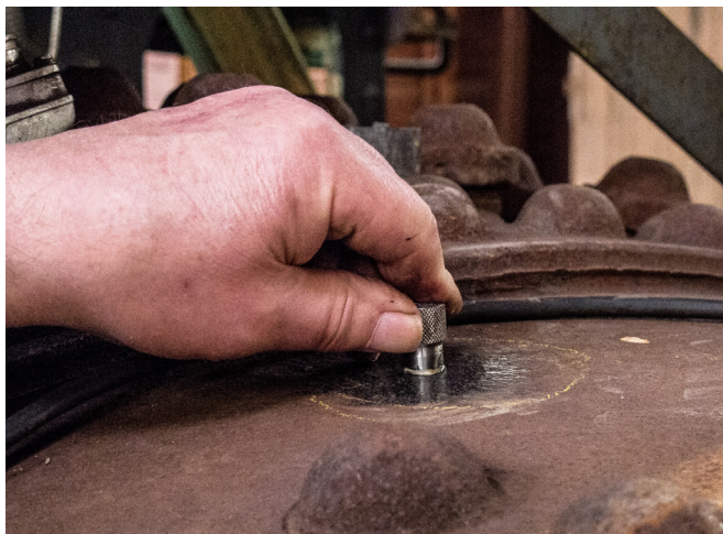
Dennis Daugherty taking an ultrasound reading on the top of the boiler. John Wright Photo
