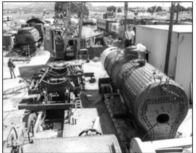
The ALCo boiler has been removed from 2353's frame (to the left) for transport to Fraser's Boiler Service, May 9, 1992. Photo by Dick Pennick
