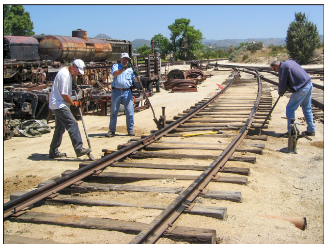
Bob Nickels, Walt Novinger and Larry Owen dig out the ballast around the ties. Photo by Jim Baker
