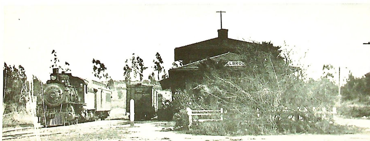
Fallbrook local, Locomotive No. 698 and combine, at "New" Fallbrook Station, about 1925. (R. P. Middlebrook picture)
