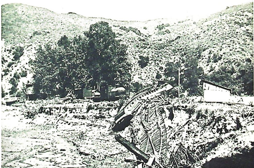
Original Fallbrook station in Santa Margarita Canyon suffered severe flood damage in January 1916. River bed was scoured to bed rock and much Santa Fe property was washed away.
