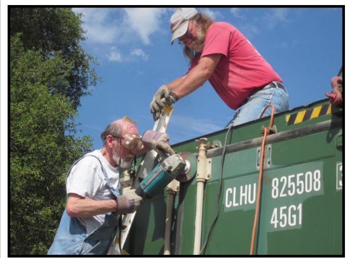
Bruce Semelsberger grinding off one of the door latches. Reena Deutsch
