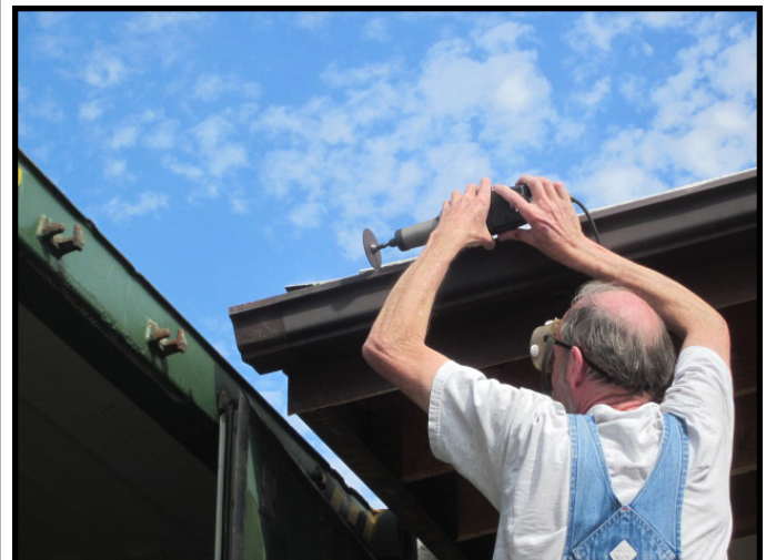
Bruce cutting off the gutter on the library roof to provide clearance for the container. Reena Deutsch
