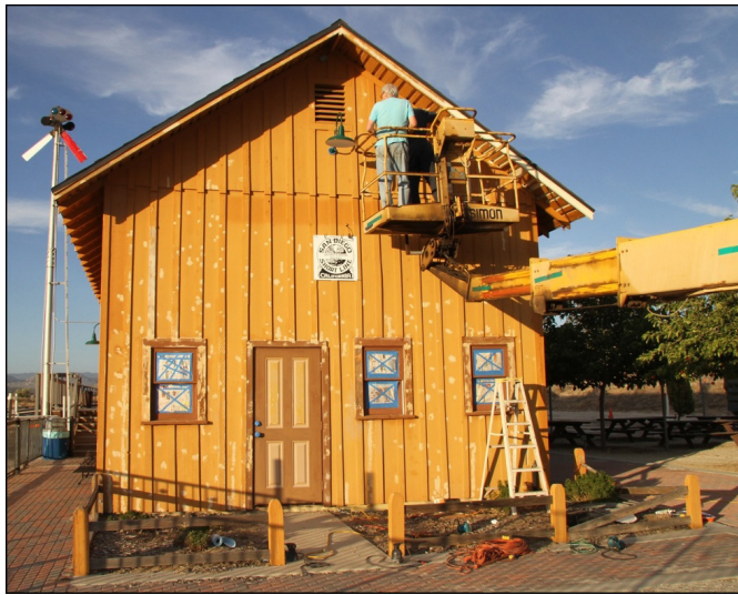
Bob Underhill (L) and Jim Lundquist up on the manlift. Photo by Frank Denison
