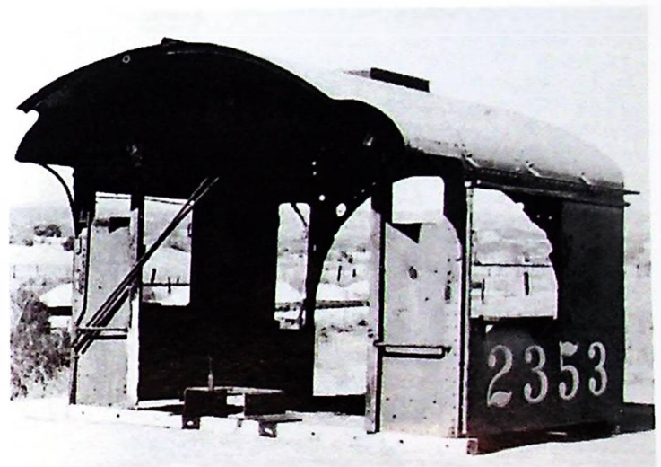
STEAM TEAM "HEADQUARTERS BUILDING" is SP #2353's cab, removed from the locomotive frame during restoration. photo-b.schneider
