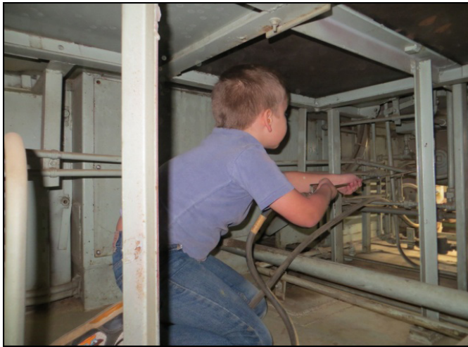
Ian Hyatt cleans out the air rack on the 7285.
