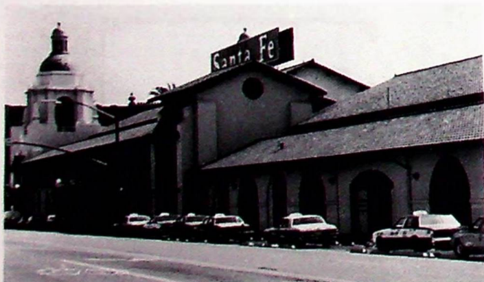
EAST SIDE of depot shows the Kettner Blvd. taxi line and its second floor. The attached baggage/express building is at the right, with the SDRM Research Library inside the shallow arch. Photo-b.schneider
