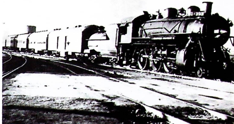
A sister to SP locomotive #2353 , #2360 departs El Centro station westbound, with the first 363 train of 6 cars. The train will soon pull out onto the main line to San Diego, and then pick up a helper engine at Coyote Wells for the uphill climb through Carriso Gorge to the Titus siding.
