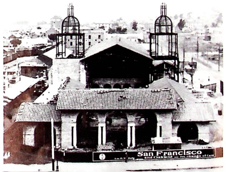
LOOKING NORTH: The Santa Fe Depot under construction on September 1, 1914. At left is the old California Southern depot.
