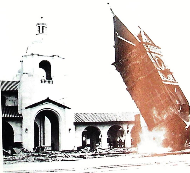
The 1887 Victorian-style California Southern depot comes tumbling down on March 8, 1915, a day after the new one was opened. Note the cable attached to two Santa Fe switch engines, and the aerial balloon overhead. Photo-an Diego Trust & Savings Bank collection.
