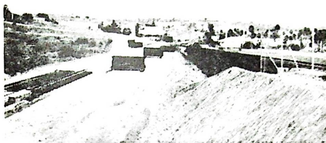
As one looks east along the La Mesa branch toward 47th Street, one sees a trestle on the right - it's probably dismantled now - and beyond it the 47th Street bridge which is now being replaced.
