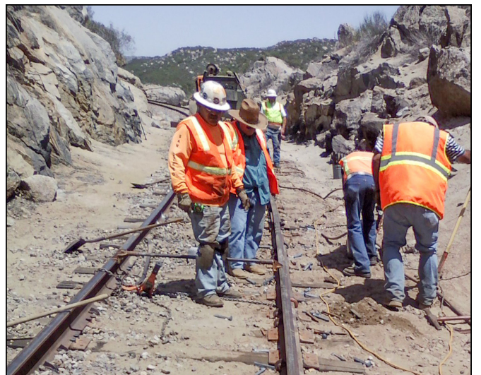
Wally Barber and his crew at work. Note the gauge bar on the track.
