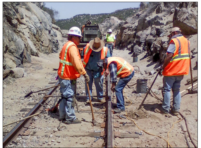
Wally Barber, in brown hat, supervises the crew working on the SD&AE right-of way.
