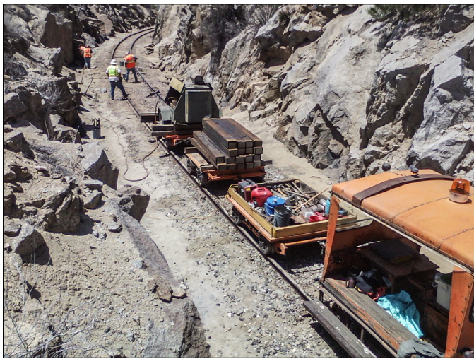
Track crew at work on the SD&AE right-of-way.
