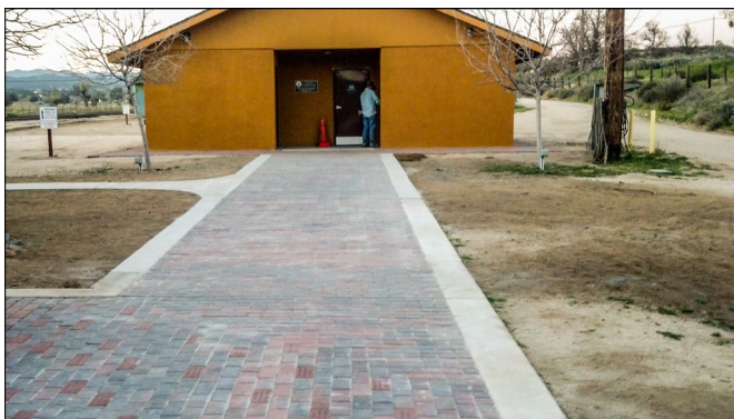
The completed brick pathway from the depot to the restrooms. Frank Denison Photo
