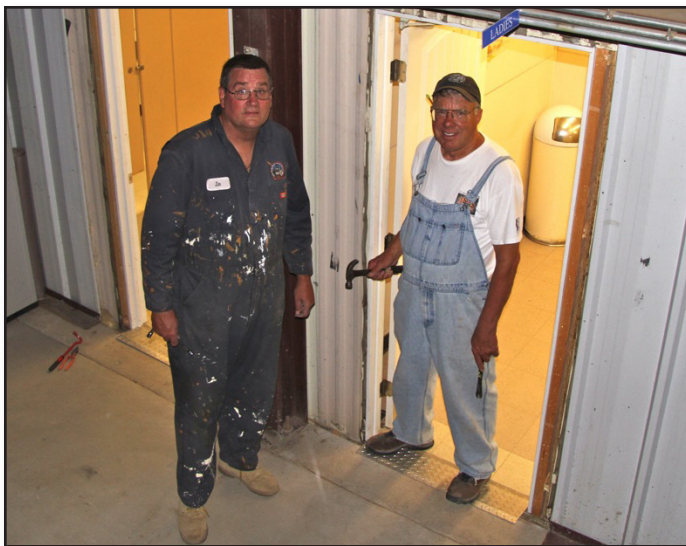
Jim Lundquist, left, and Frank Denison working on the doors to the Display Building rest rooms.
