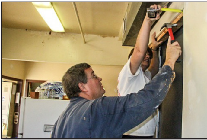
Jim Lundquist (L) and Dawn Robertson at work on the improvements to the Campo lunchroom area. Frank Denison
