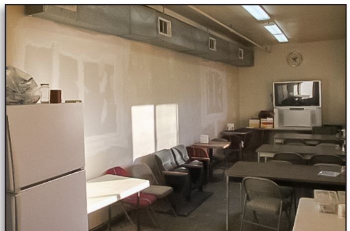
The Campo lunchroom area, showing improvements in work.
