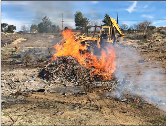
Jim Lundquist (background on the back hoe) handling the burning of debris on the PSRM property. Frank Denison
