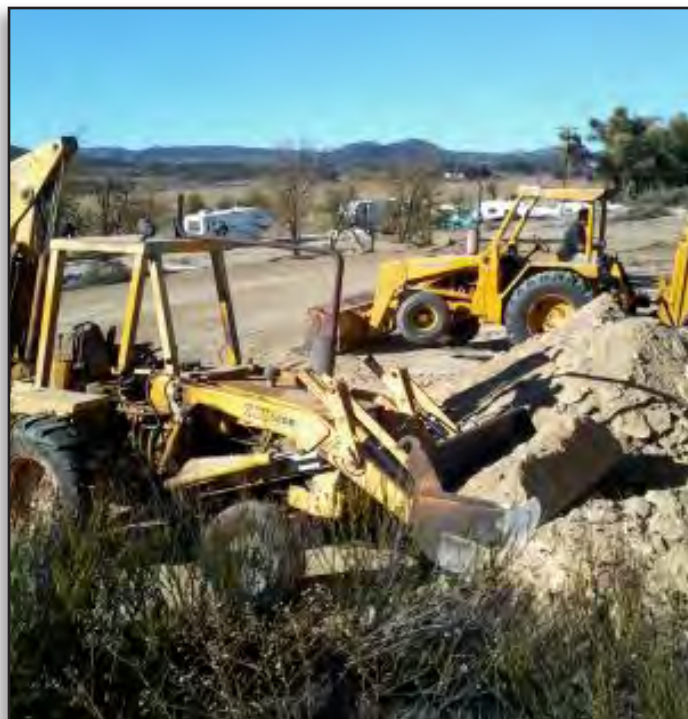
Another project taking place at Campo is the grading and leveling of a new Workamper pad. Here a contractor is working on the grading portion of the project. Glen Rogers
