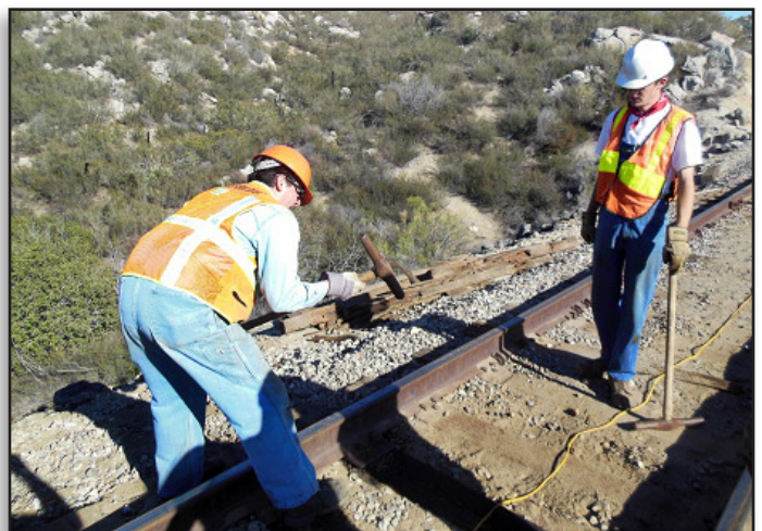
Hector Gonzalez, left, and Martin Caestecker take turns spiking down the rails.
