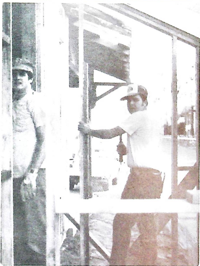
Jim Lundquist, later President and first Executive Director of the Museum, and Larry Rose, its General Superintendent, architect, and REPORT editor, work on rebuilding the La Mesa Depot in June 1980.
