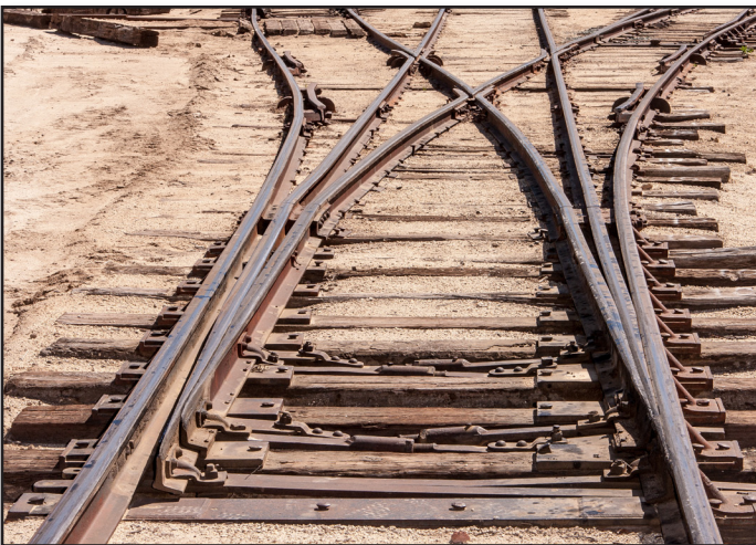
The rare three-way switch in the Campo yard.
