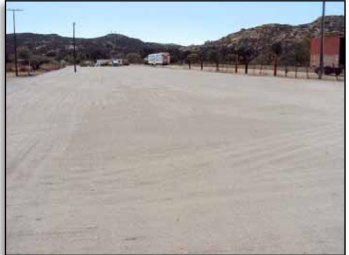
The completed parking lot resurfacing project completed. Dave Tomeraasen
