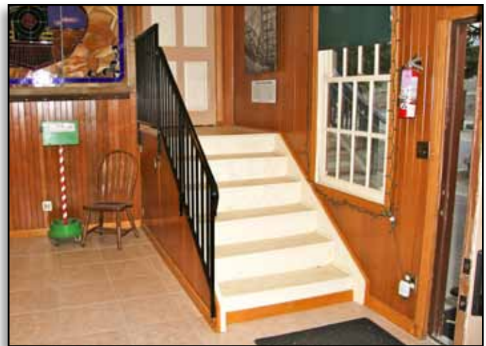
A new railing has been installed on the stairs from the Gift Shop to the waiting room at the Campo Depot.
