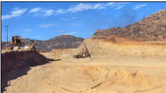
The work on the daylighting of Tunnel 3 in Mexico is progressing. Dave Tomeraasen
