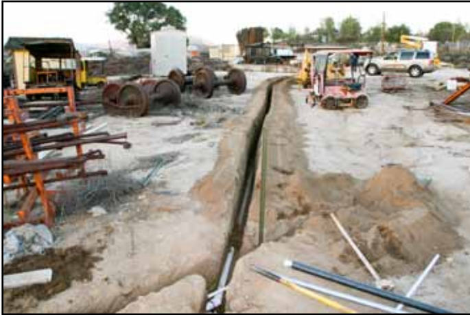
The trench with piping place for the water line to the library. Frank Denison
