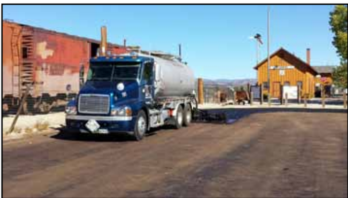
Oil being applied to the parking lot at the Campo Depot. Frank Denison
