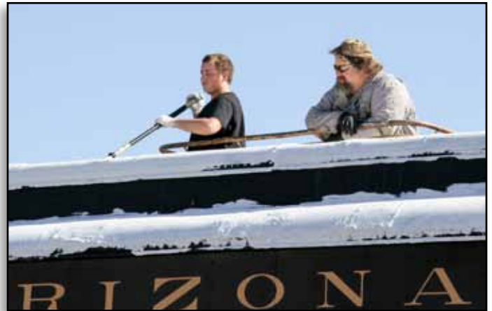
Cary Hyatt and Robbie Smith waterproofing the roof of one of the coaches. Frank Denison
