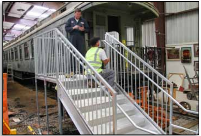
The almost-completed installation of stairs for access to the SD&A 050 car.
