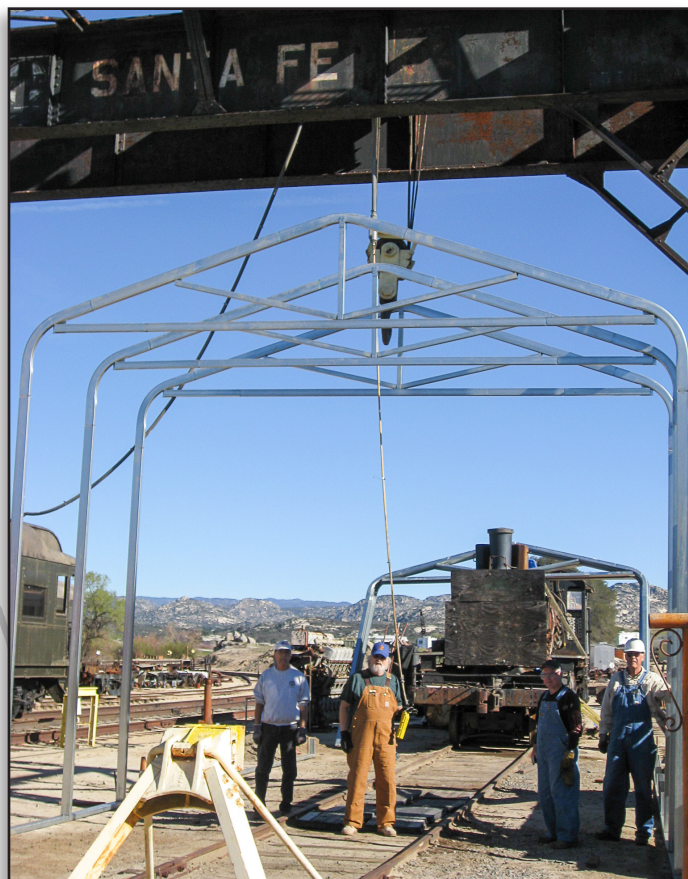
Hoisting the frames into place; Bob Nickles, John Wright, Harry Lineback, Rich Paulus. Jim Baker
