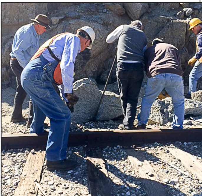
MOW personnel remove a large rock from the right of way. Harry Lineback
