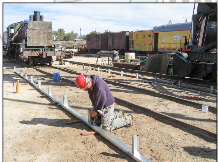
Mike Lucek drilling tie down holes in the west base rail. Jim Baker
