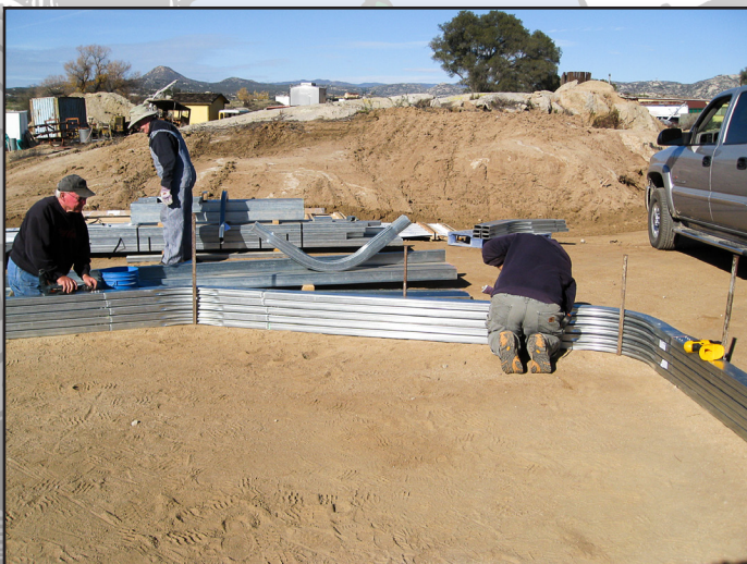
Harry Lineback, Ron Amberger, and Mike Lucek working on the wall/roof frame assemblies. Jim Baker
