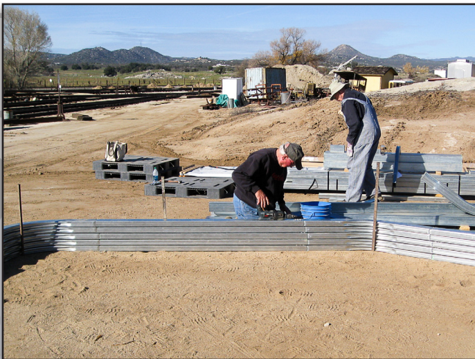
Harry Lineback and Ron Amberger working on the wall/roof frame assemblies. Jim Baker
