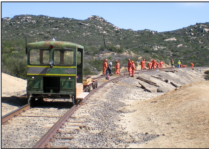
PSRM gang car and CalFire work crew replacing ties. Glen Rogers
