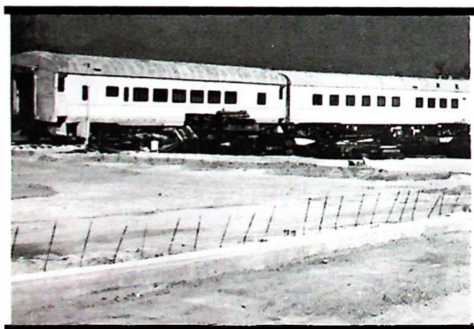
Footings for the new building at Campo are seen in this March 11th view. In background are UP coach #576 and cafe car #4054.
