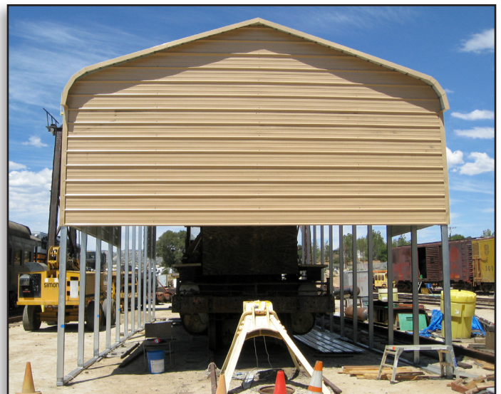
Completed West end.
