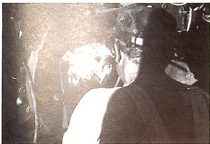
Fred Perry watches the flaming waste fire starter to observe the blower adjustment before moving it down in front of the burner to ignite the oil.
