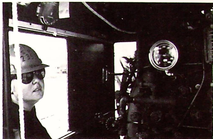
Karla Von Huben takes a turn at the firing controls. The team tested all steam boiler controls including the blow-downs, injectors, turret valves and the throttle.
