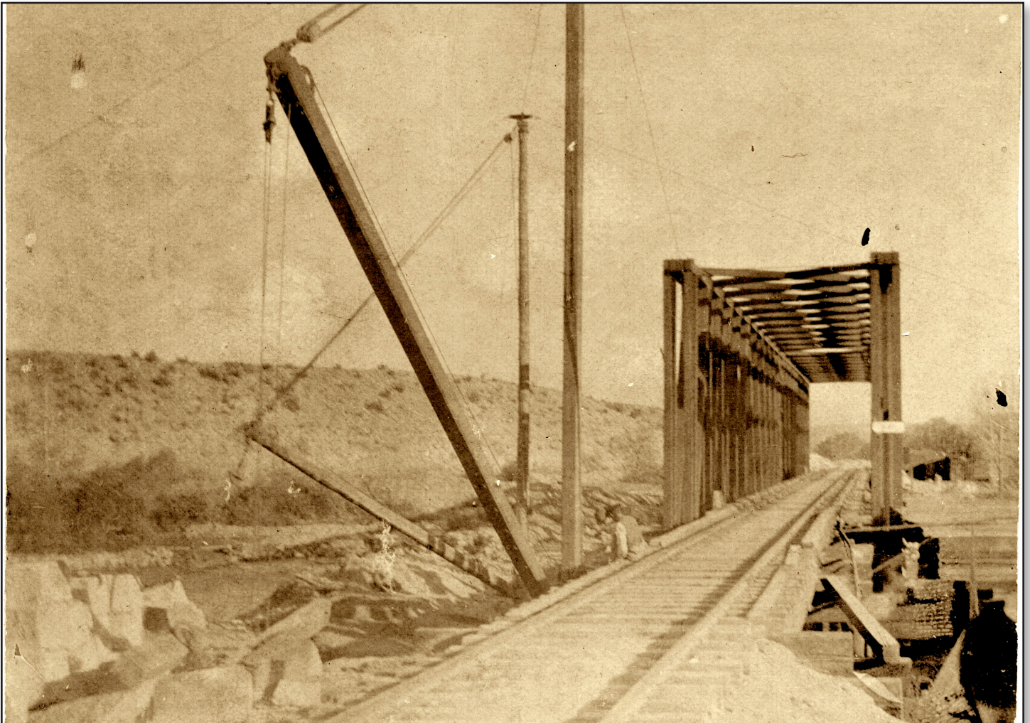
A railroad bridge in Pueblo, Colorado ca 1901. This bridge was built by the Colorado Fuel and Iron Company and W. H. Glascock, a long time railroad worker was part of the construction crew. An article on the W. H. Glascock donation to the museum library begins on Page 2.
