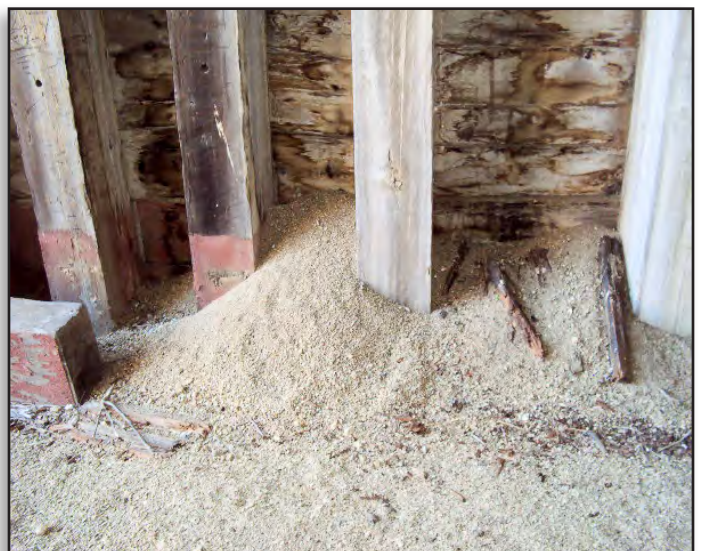
Closeup of the erosion at the west portal of tunnel 4.
