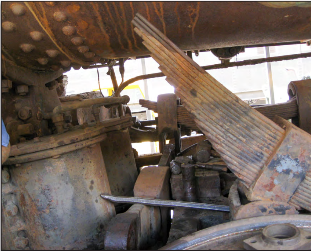
The left front spring with the pin and front hanger removed.
