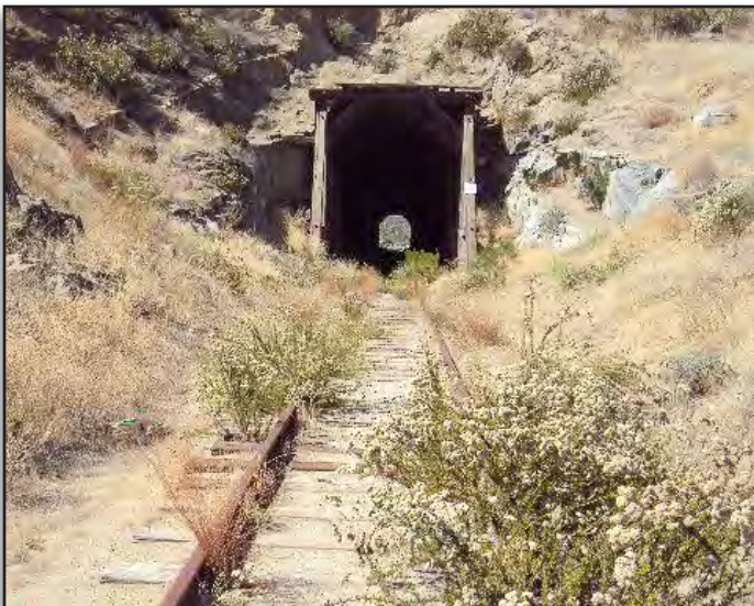
Tunnel 4, west portal looking east towards the United States.
