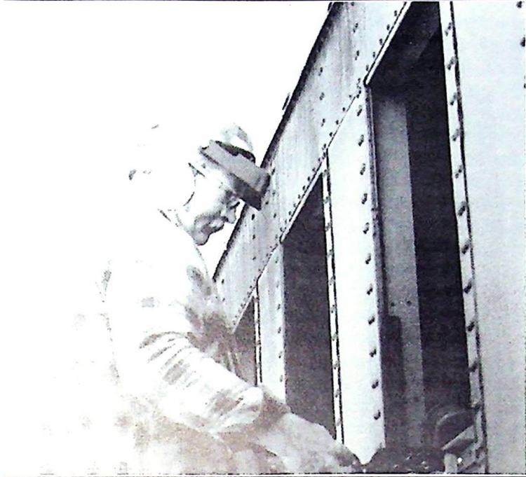
Jim Campbell installing new window sills on Santa Fe RPO 74 December, 1995.
