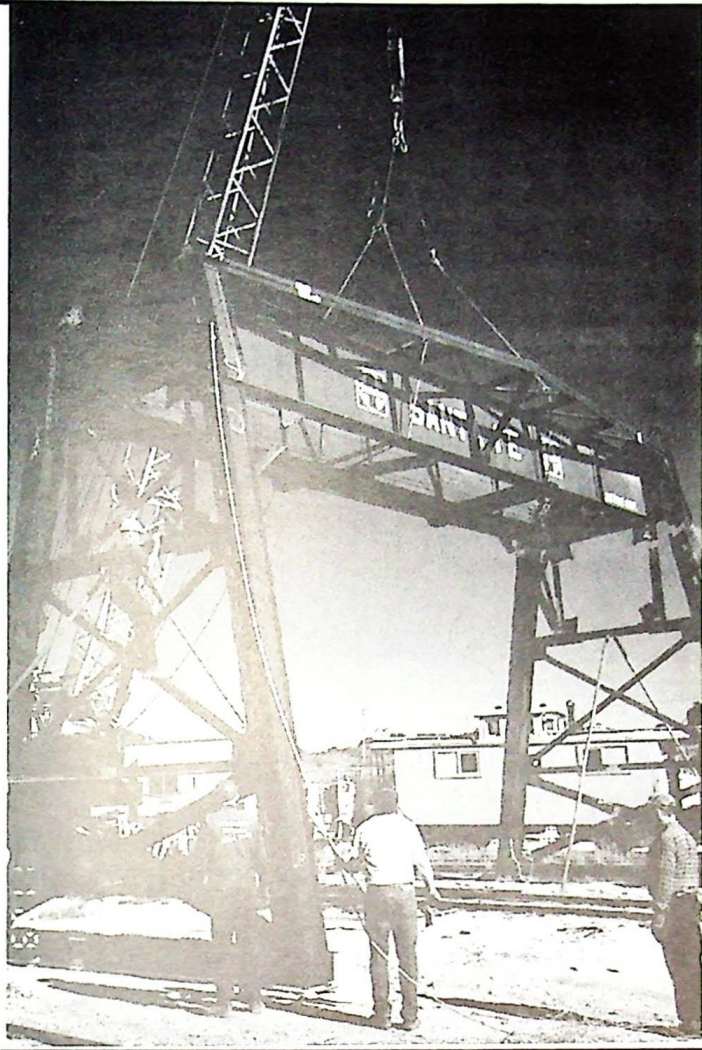
Dick McIntyre climbs up to secure our rolling gantry crane to its legs as Richard Dick, Paul Westover and Bob Haney watch.
