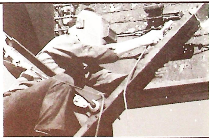
Dick McIntyre thirty feet in the air welding the crane back together piece by piece, just as he cut it apart in San Diego 11 years ago. An amazing craftsman and an amazing job!
