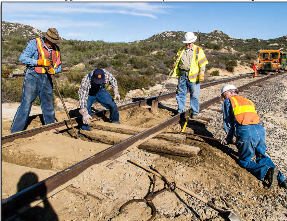
Dick Pennick, William Crawley, Glen Rogers, and Rich Paulus replace several worn ties along the right-of-way. John Wright
