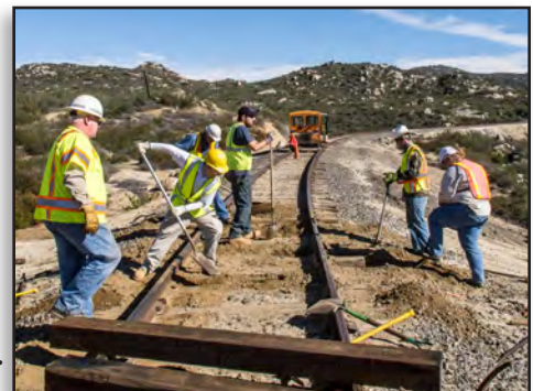
Glen Rogers supervises a crew replacing ties along the right-of-way. John Wright
