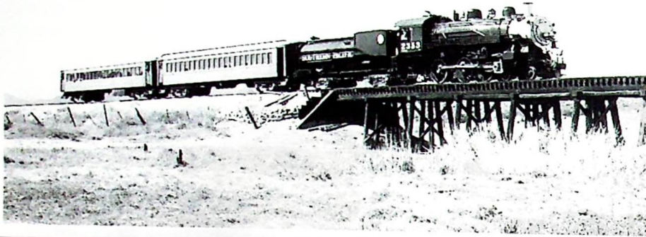
SP #2353 and short passenger train crosses pile trestle in a pastoral setting just east of Campo on March 2, 1996. Short shuttles behind the steamer were run all day for visitors as part of the "First Rollout" ceremonies. The old engine performed flawlessly as it recreated its original role as a passenger hauler.
