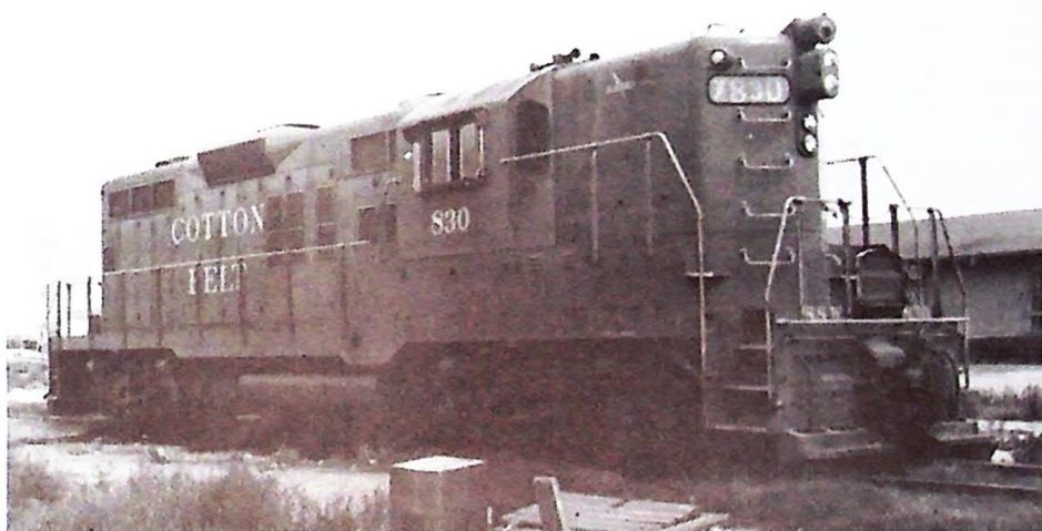
St. Louis Southwestern (Cotton Belt) #3873 is shown here in its original Scarlet & Gray colors as SSW #830 in Brownsville, TX on June 24, 1962. The EMD GP9 diesel-electric was built in 1959, rebuilt in 1977 and is similar to GP9's used by the SP on the SD&AE. Note the small cab numbers characteristic of SSW units, pilot beam lettering, lightning bolt "Radio" stencil and lights. It has dynamic brakes and MU capability.
