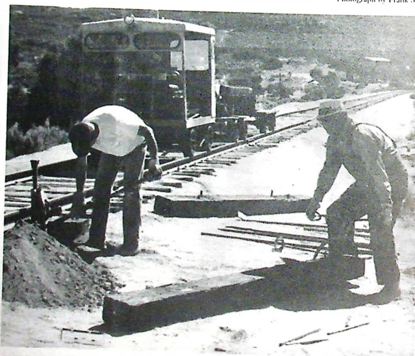
Kevin Dudenbostel (left) and Allan Dillane (right) are shown working on the Museum's tie replacement program on inaugural day June 29, 1996.
