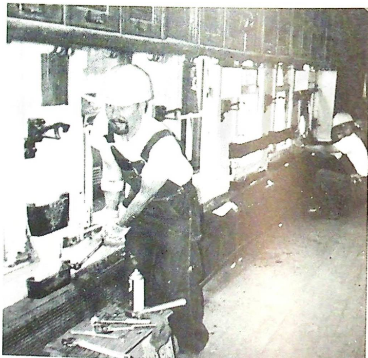
Restoration Superintendent Ted Kornweibel and Frank Stites work on RPO #74's hardware and windows in August, 1995. Repairs and replacements were badly needed!
