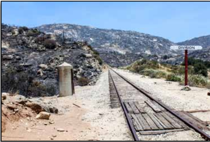
The concrete telephone booth and Division station sign remain untouched amid the charred countryside.
