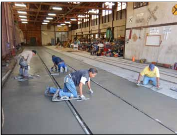
Brian Elmore and his crew finishing with the concrete pour in the shop building.
