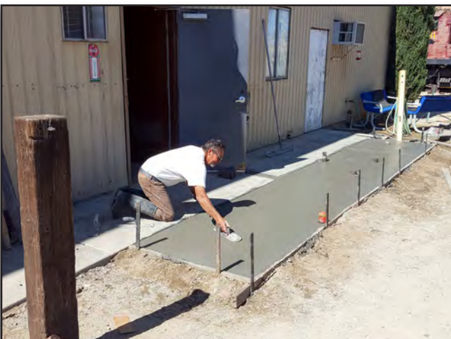
Brian Elmore works on the concrete for the wind break at the shop building. Jim Lundquist
