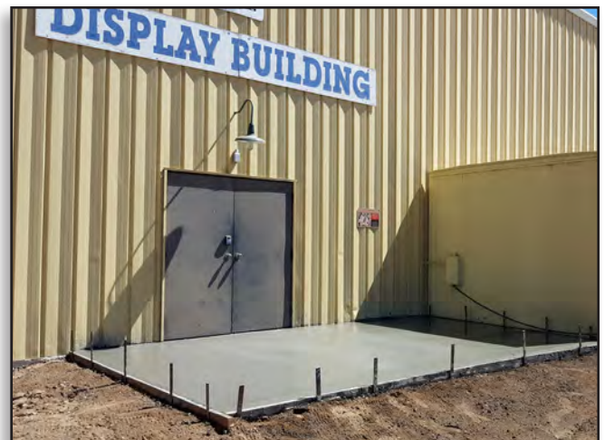
Concrete pad poured for the wind brake at the Display Building. Jim Lundquist
