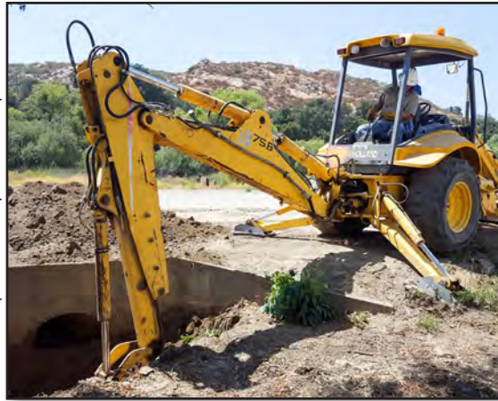
Glen Rogers using the backhoe to clean out one of the drainage culverts on the museum property.
