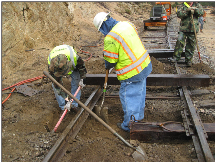
James Caestecker and Glen Rogers digging out a space for a new tie. Jim Baker
