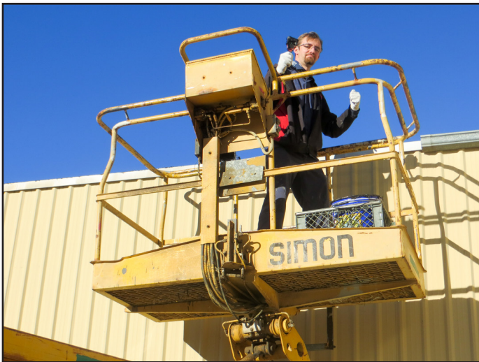
Martin on the man lift accessing the roof of the Car Shop. Ron Hyatt
