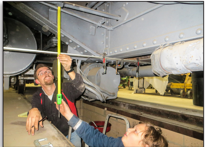
Martin and Aaron take measurements from the undercarriage of UP 576 for future waste tank.
