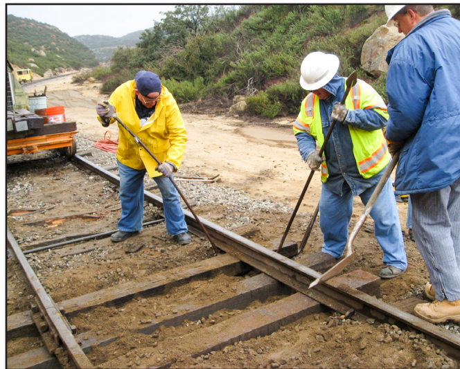
Jim Peterson, Glen Rogers, and Jim Lundquist doing initial tamping of new ties. Jim Baker
