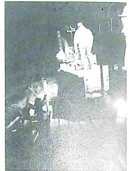
Work continued late into the night in order to have things ready for the April 26 trip.
