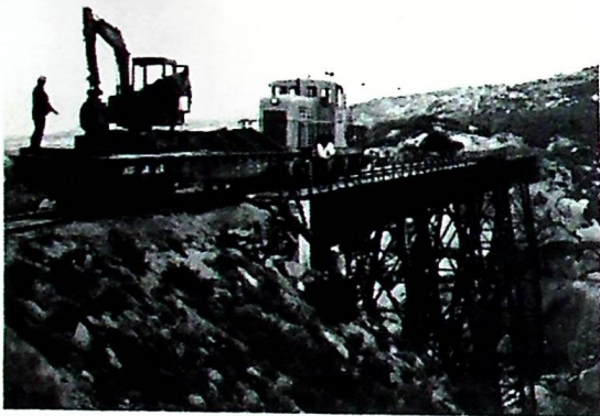
Several days before the trip, a final work train ran to do repairs at the high bridge. Museum's #7285 doing the honors and Benny Wright working his magic to fix the track.
