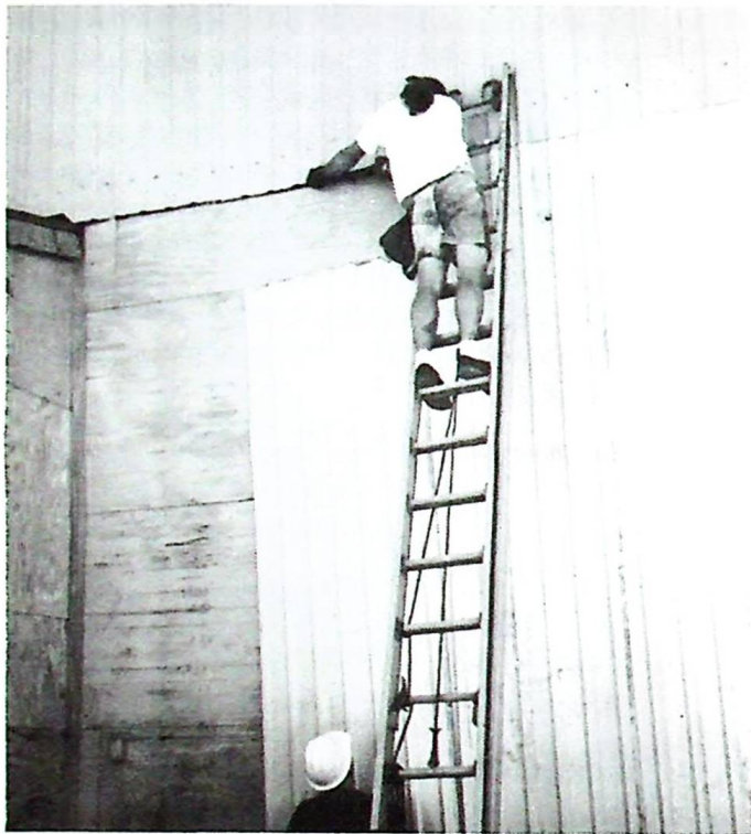
Tom Clark and Randy Gibson completing the siding to the car barn.
