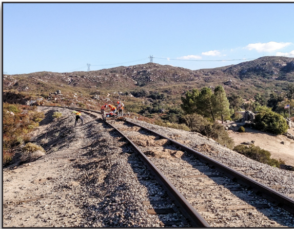
Hand crews dress and spike the track ahead of the Tamper.
