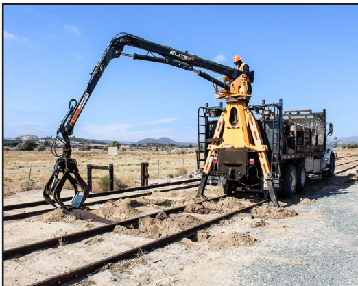
The Grapple Truck inserts a tie near the west end of the Campo siding.
