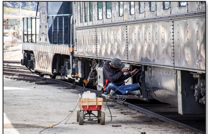
Martin Caestecker services the batteries on the Robert Peary.
