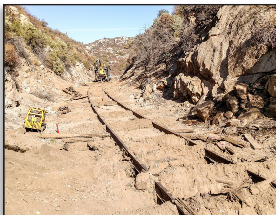
In the distance, the Grapple Truck inserts ties in the MP 63 cut after the backhoe has removed the old ties.
