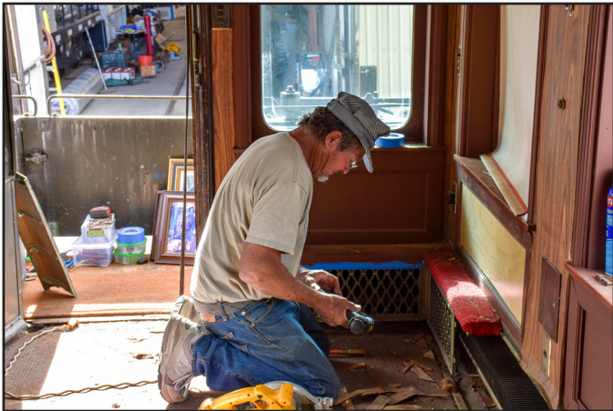
Brian Elmore works on installing new carpet in the Robert Peary's solarium.
