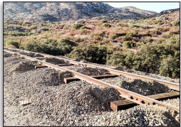
Ties waiting to be tamped just east of MP 63.
