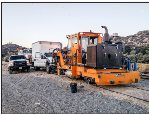
The Tamper and Welding Van are refueled on the House Track early in the morning.
