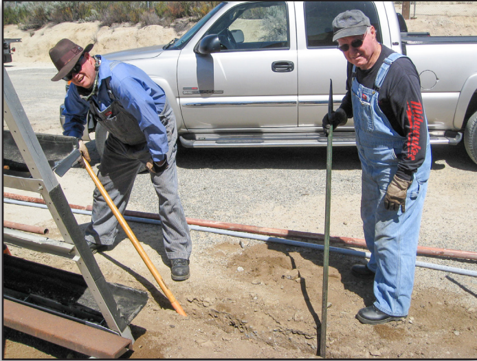
Tim Wamsley and Harry Lineback digging the trench, Campo, May 11, 2018. Jim Baker
