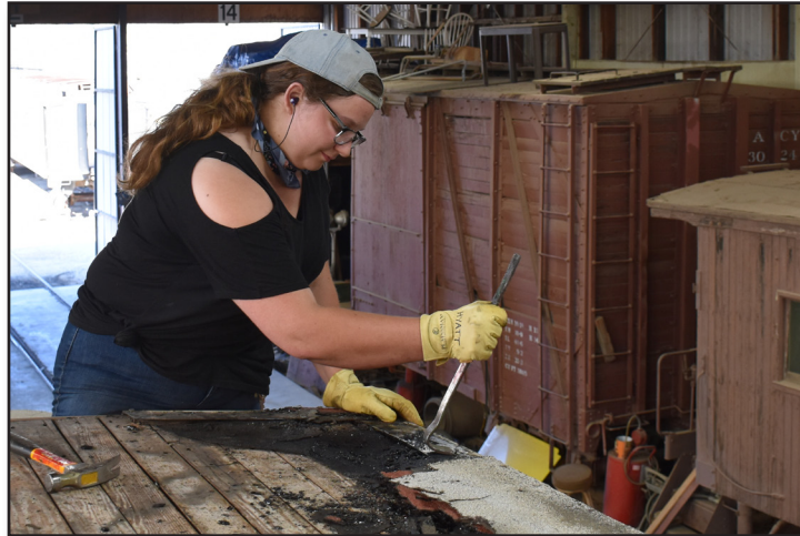
Alanna Hyatt works on removing layers of roofing on the C&O caboose. Diana Hyatt
