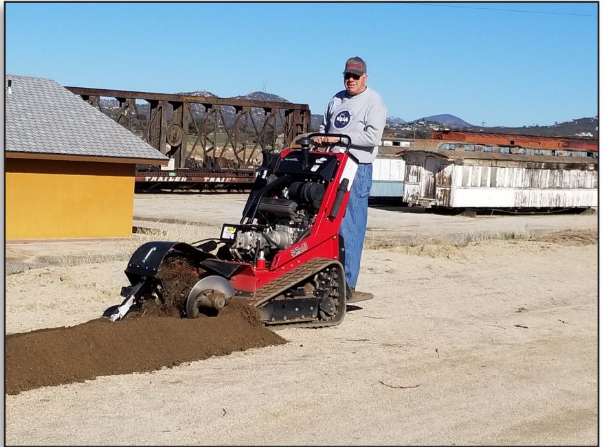
Frank Denison is on the tracked trenching machine installing new water pipe on January 10, 2019 Jim Lundquist
