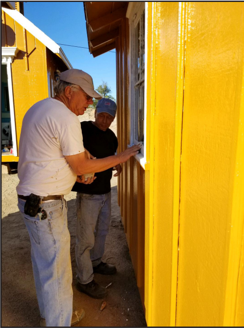
Frank Denison and Steven Pohjola working on the DAP Depot at Campo. Dawn Lundquist
