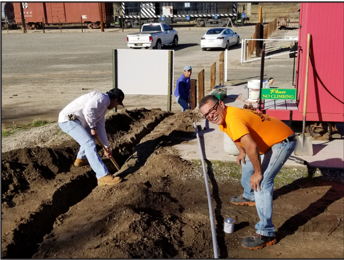
Dan Cottado, Steven Pohjola and Adolfo Rico are installing conduit and water lines for the DAP Depot on January 10, 2019. Jim Lundquist
