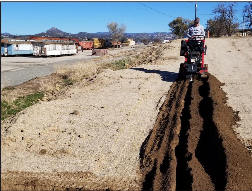
Frank Dennison is on the tracked trenching machine installing new water pipe on January 10, 2019 Jim Lundquist
