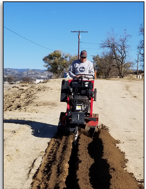
Frank Dennison is on the tracked trenching machine installing new water pipe on January 10, 2019 Jim Lundquist
