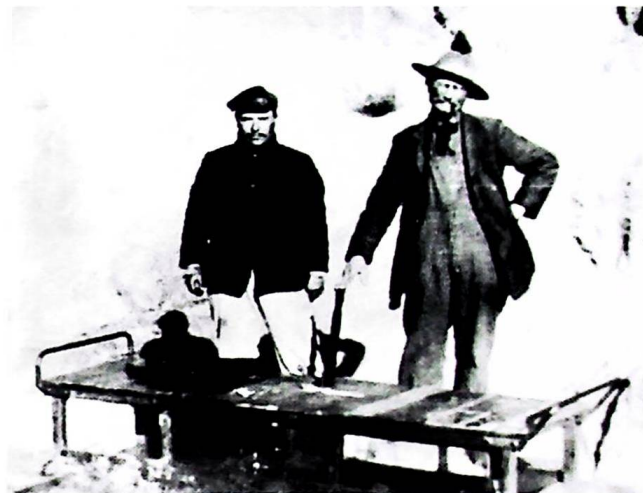
Edmund Kallright (right) poses with the motor car operator somewhere in Mexico during construction of the SD&A about 1915. Photo is from the Lloyd Norris (former SD&A locomotive engineer) family scrapbook at the Bonita Museum.
