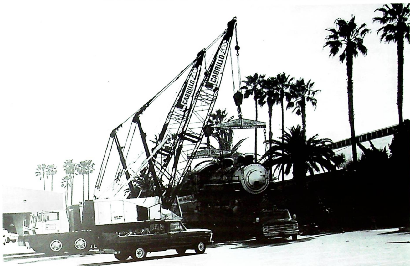
Two large cranes do a "clean and jerk" lift of our 100 ton Baldwin product at the Del Mar Fairgrounds on Feb. 15, 1983. The engine is being placed on house moving dollies for the two mile move to the Solana Beach Lumber Yard spur. From here it would go on it's own wheels all the way to our Museum at Campo, altogether about 85 miles. Larry Rose Photo.
