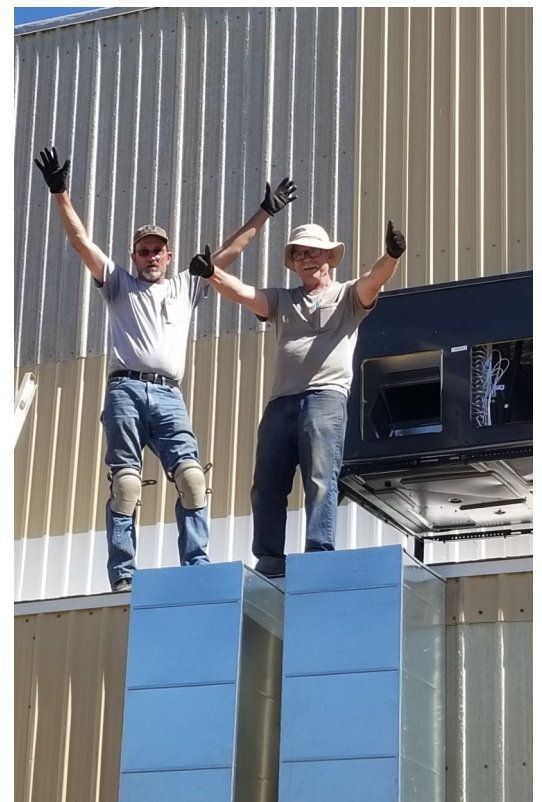
Quick Response A/C completes the A/C install for the lunch room
