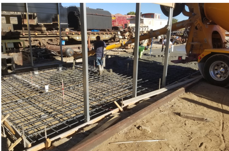
Rebar and preparations are ready for concrete pour
