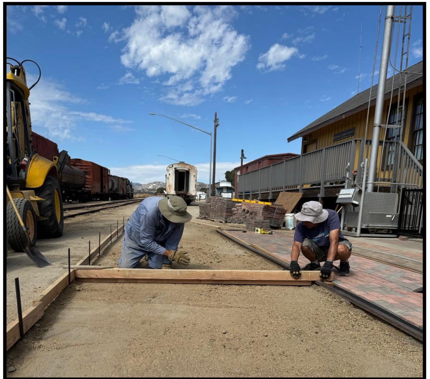
(left) Steve runs the vibrator packing down the DG.
