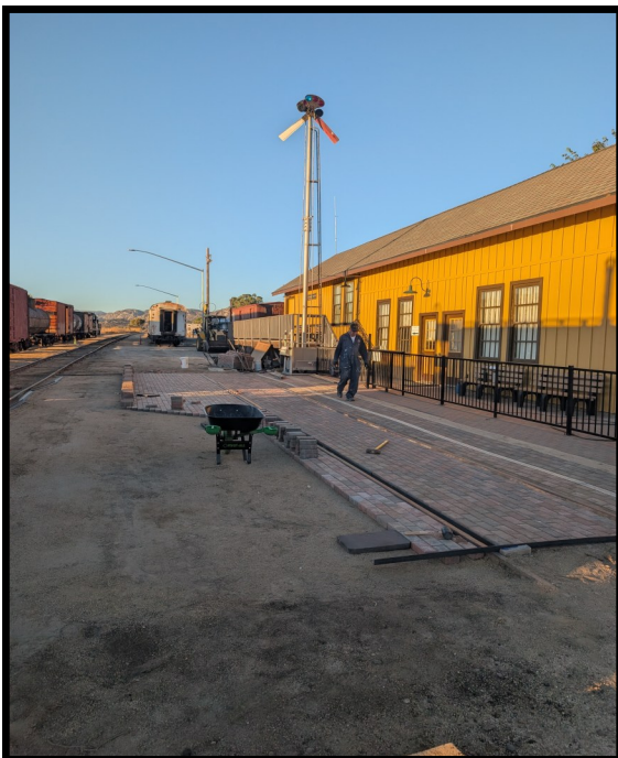
(Above) Jim and Steve level the DG.
