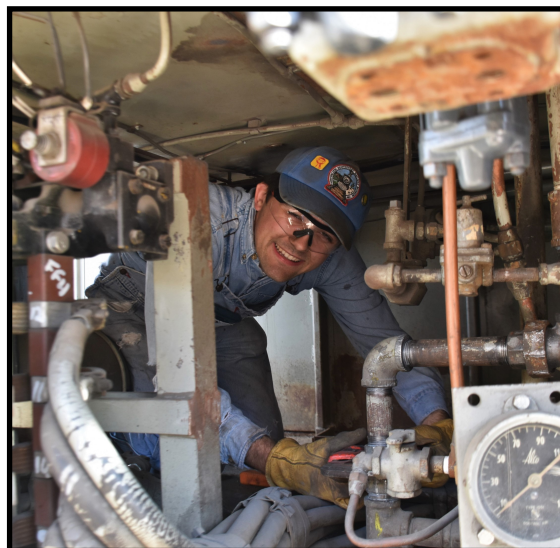
Cover photo Stephen Hager tests the GE 70-tonner for air leaks
