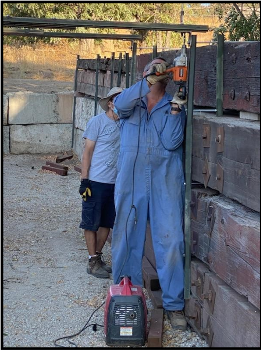
Jim Lundquist with Steven Pohjola installing braces on the Athey Mine at Campo. The mine will feature a roof and be used to keep the mine train out of the weather when completed.
