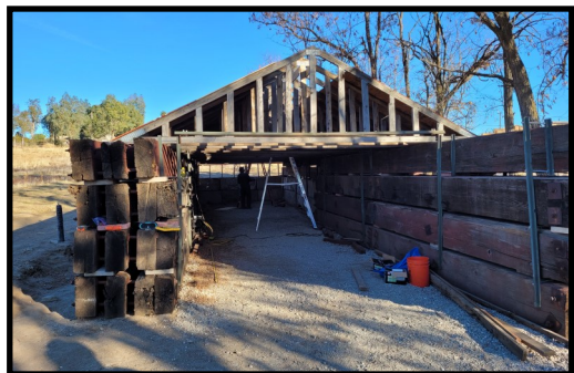
Mine train building gets a roof
