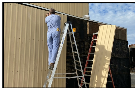
Jim Lundquist applies paneling to the side of the car shop
