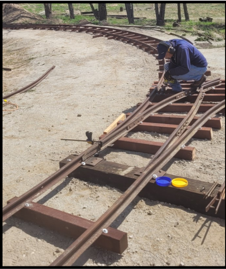
Steven Pohjola laying tracks for the mine train.
